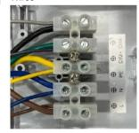
Make sure to use only Dim - & Dim + signal wires in right position
